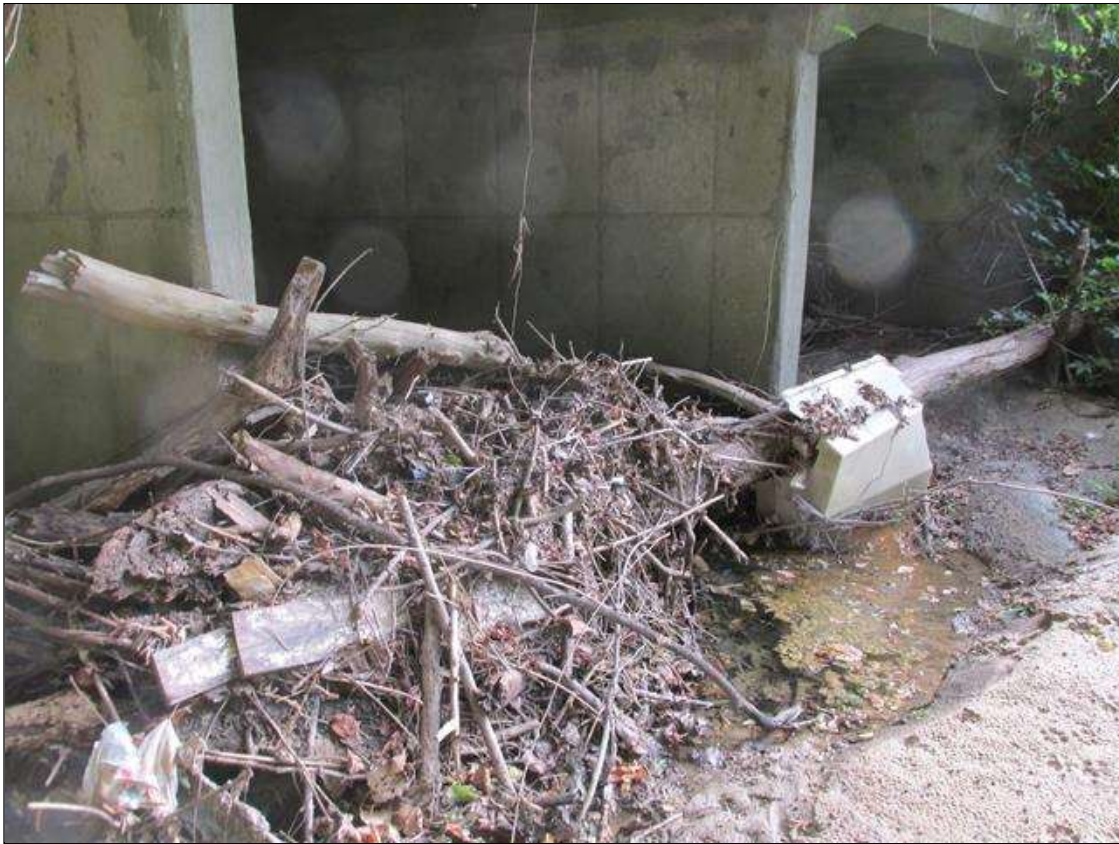
DRIFT COLLECTED ACROSS BARRELS 2&3, UPSTREAM END
