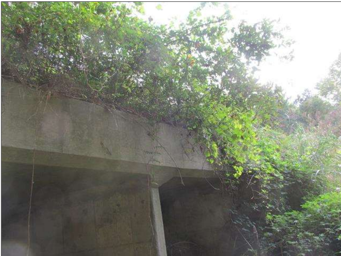
VEGETATION ALONG HEADWALL AND WINGWALLS AT UPSTREAM END
