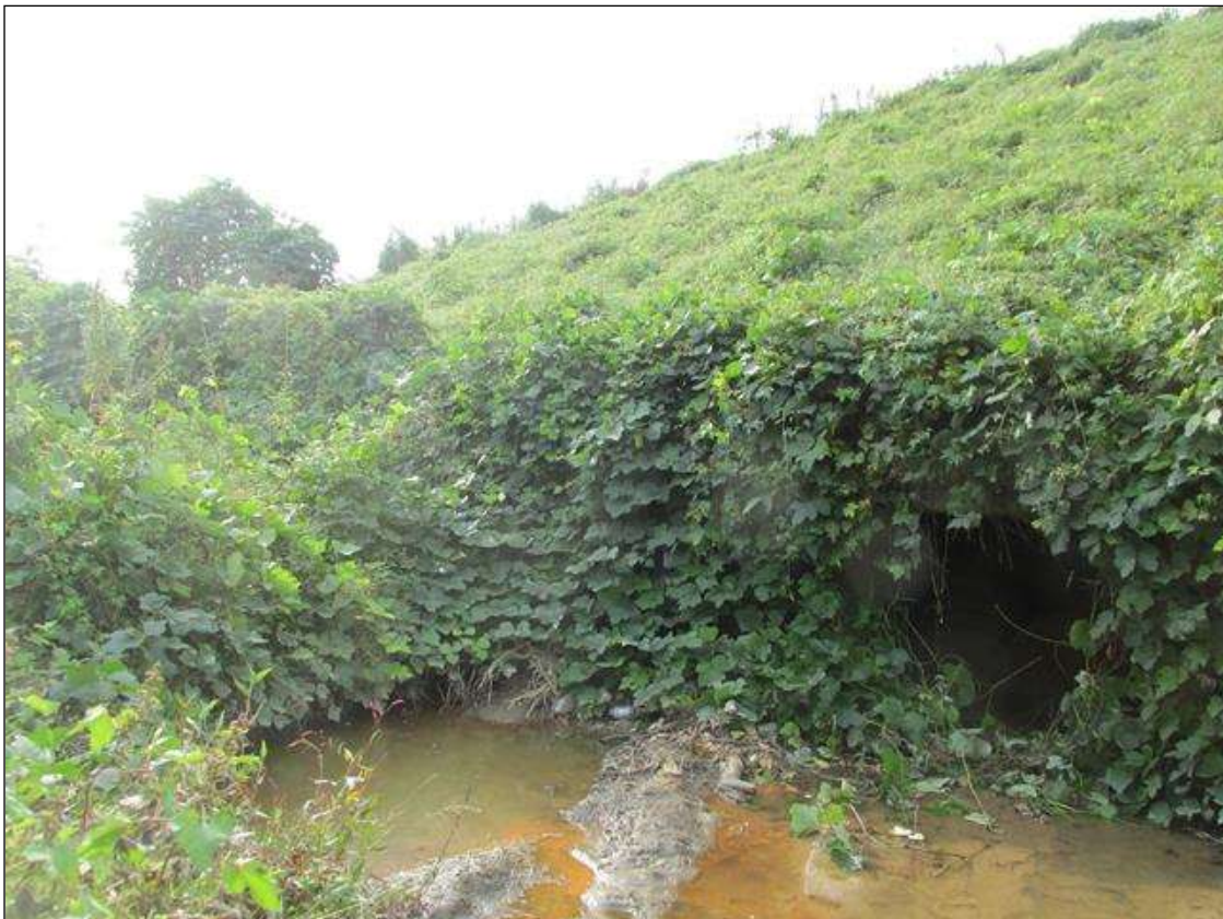
VEGETATION GROWING ALONG HEADWALL AND WINGWALLS, DOWNSTREAM END
